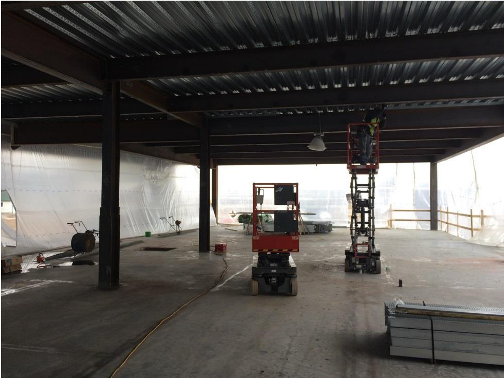
Top track being installed in sequence 1 2 nd level
