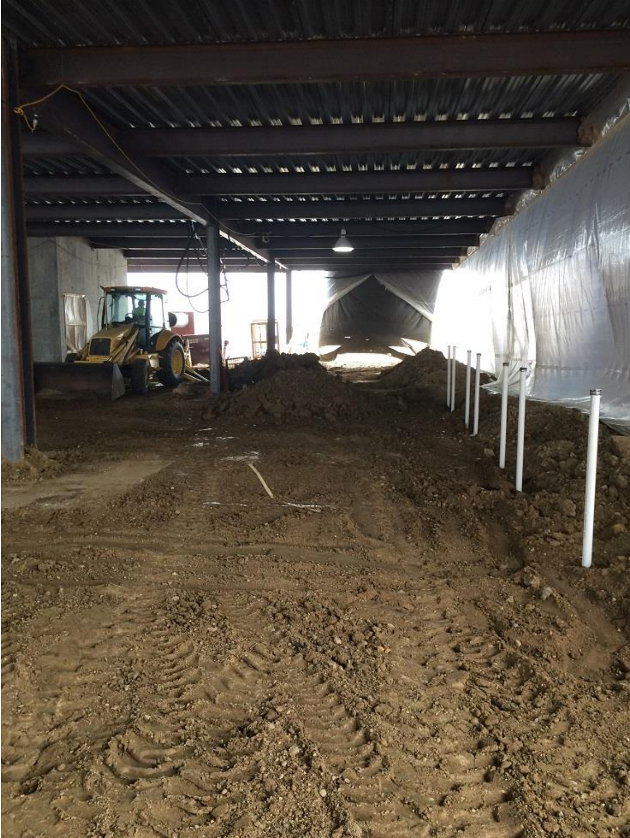
Underground plumbing progress in sequence 1
