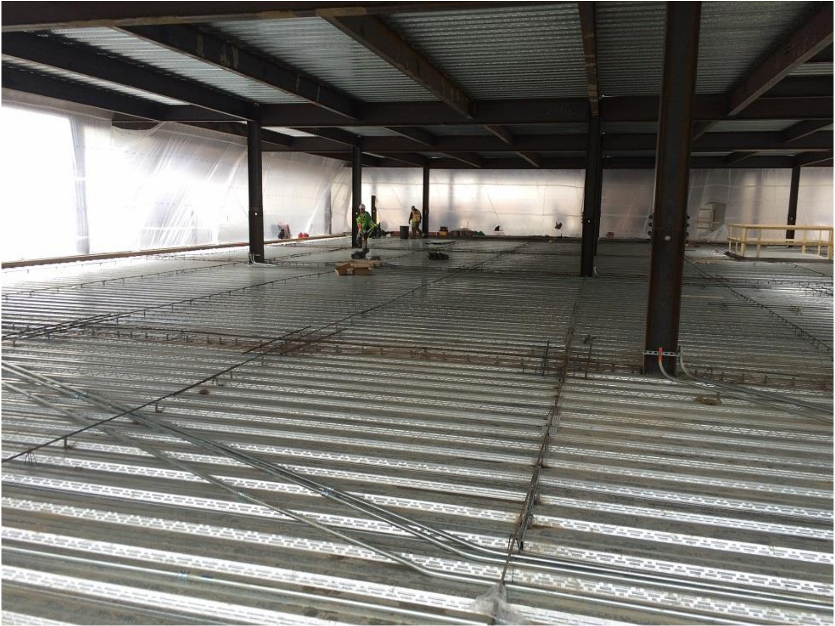
Decking complete and electrical conduits being placed on 2 nd floor deck
