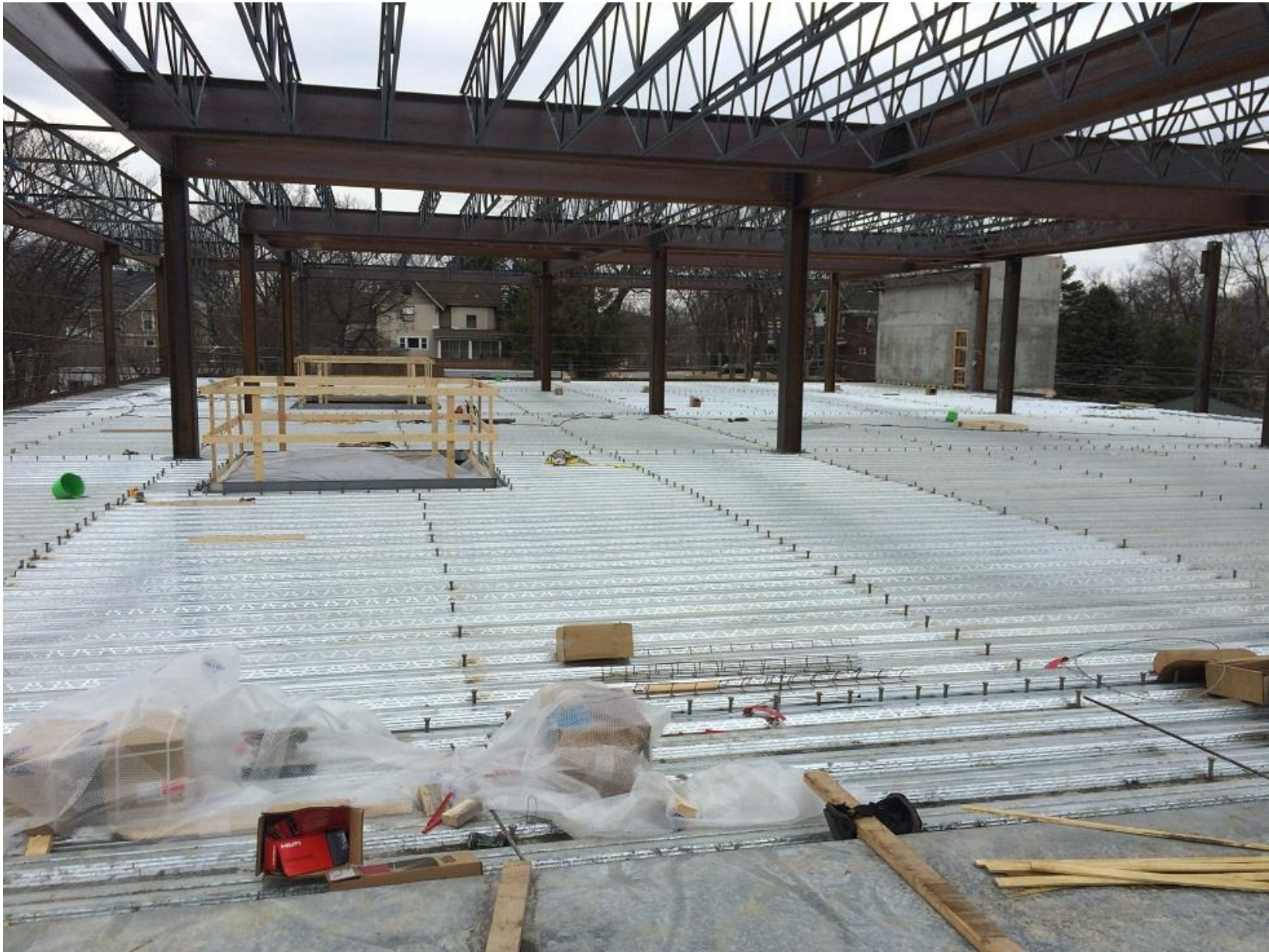
Decking installed on 3 rd level sequence 2
