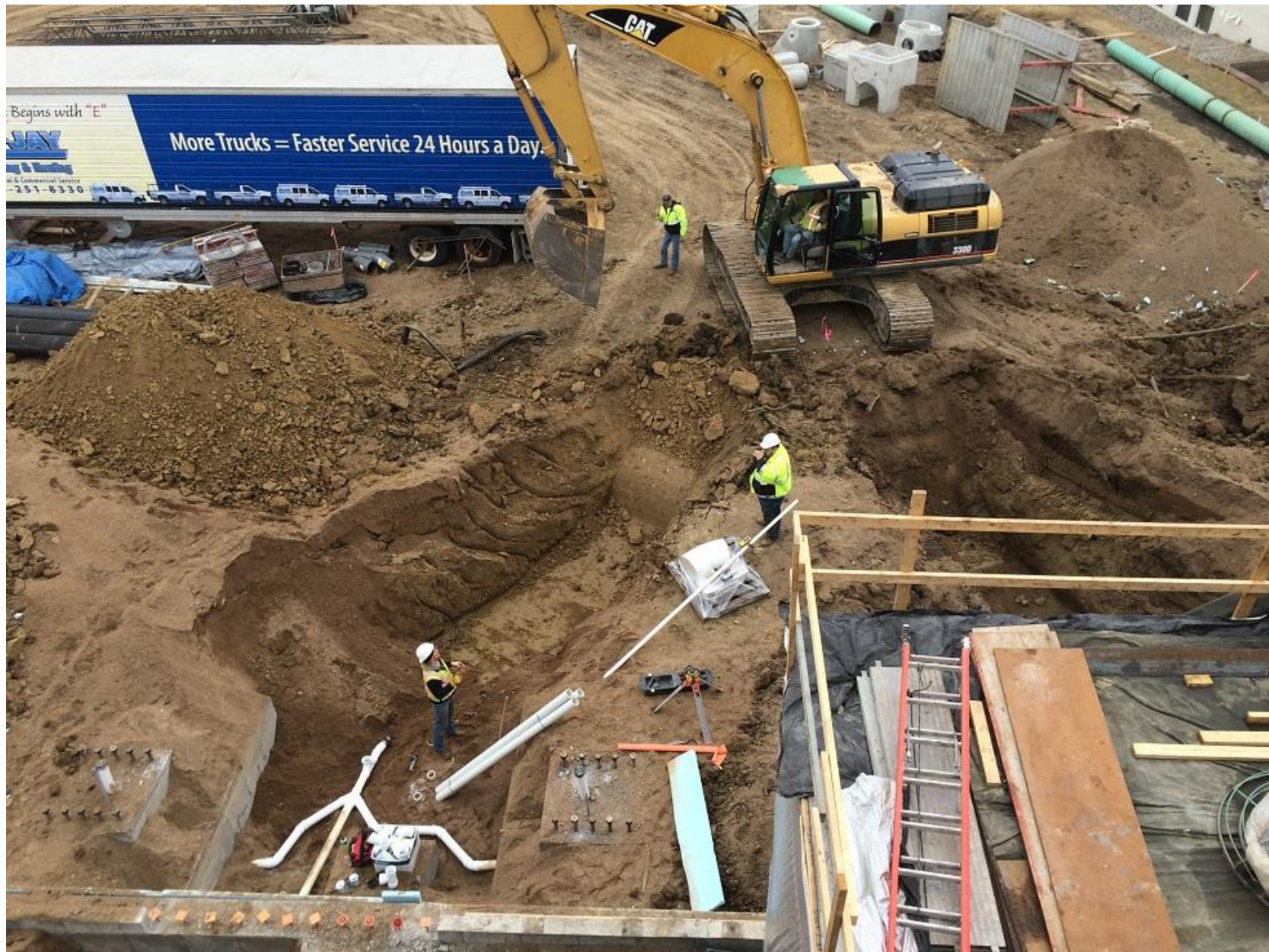
Site utility tie ins on north side of new clinic
