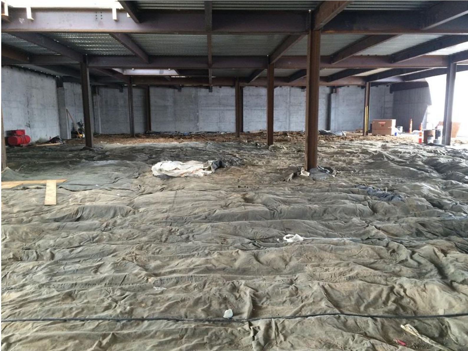
Ground covered in sequence 2 in preparation for underground plumbing
