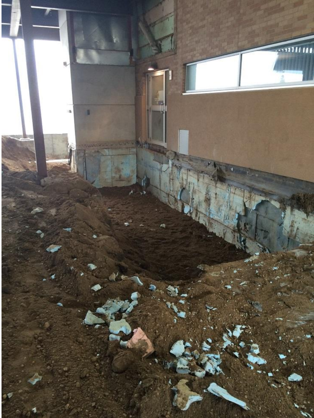
Footing trench along existing hospital
